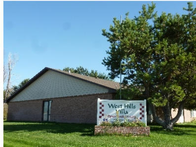
WEST HILLS 610 Pine Street
